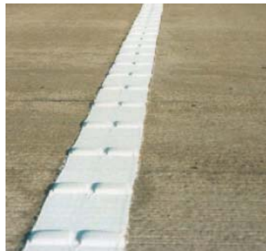
Figure 5.7: Raised ribs across profile linemarking
