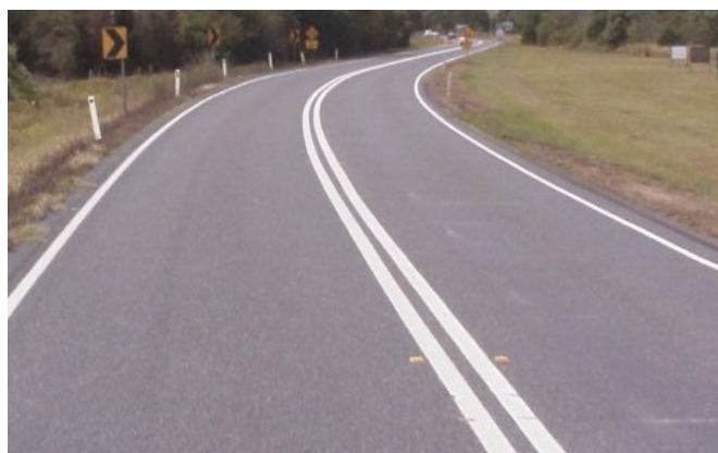
Figure 5.3: Enhanced dividing (barrier) line (BB1)
