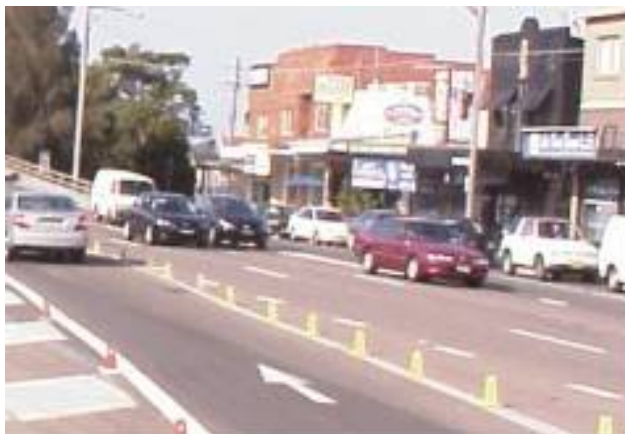
Figure 5.11: Enhanced lane separation devices (Pavement flaps)
