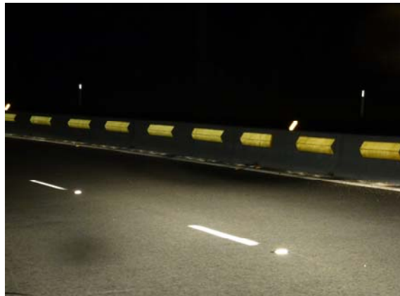
Figure 5.21: Application of enhanced Safety Barrier treatment – Central Concrete Barrier
