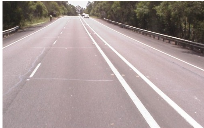
Figure 5.4: Enhanced dividing (barrier) line (BB2)
