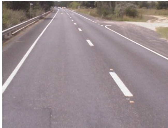
Figure 5.1: Enhanced dividing (separation) line (S3)
