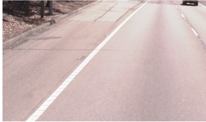
Figure 5.8: Type A Profile linemarking
