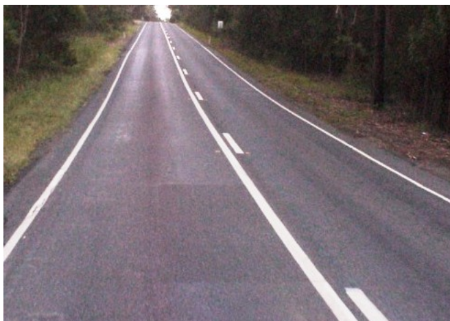
Figure 5.2: Enhanced dividing (barrier) line (BS1)
