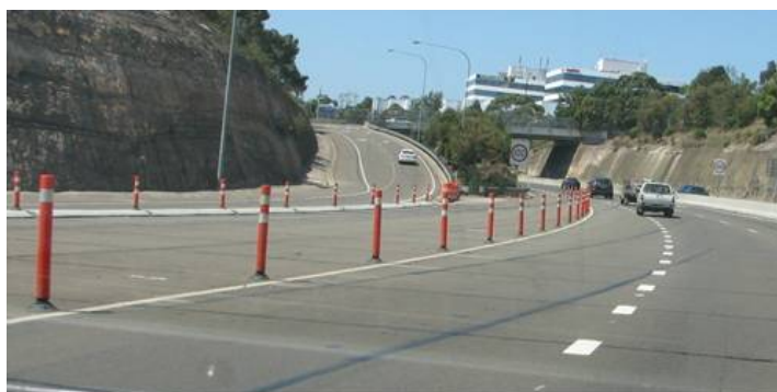
Figure 5.13: Enhanced lane separation devices (Flexible bollards)
