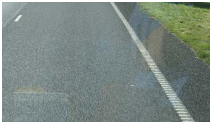
Figure 5.9: Type B Profile linemarking
