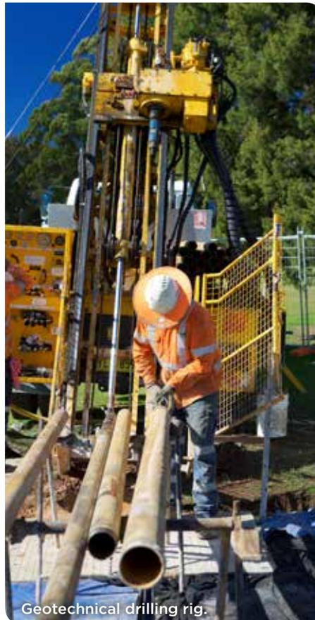
Geotechnical drilling rig.
