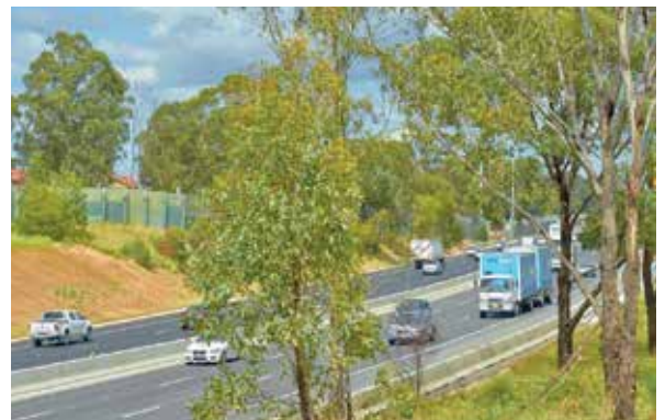
Three lanes open in each direction near Liverpool
