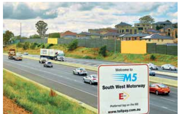
New noise wall panels installed in Prestons
