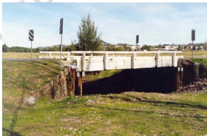
**Figure 6.2.3-1 Typical Shire Bridge Timber Kerb and Rail**
