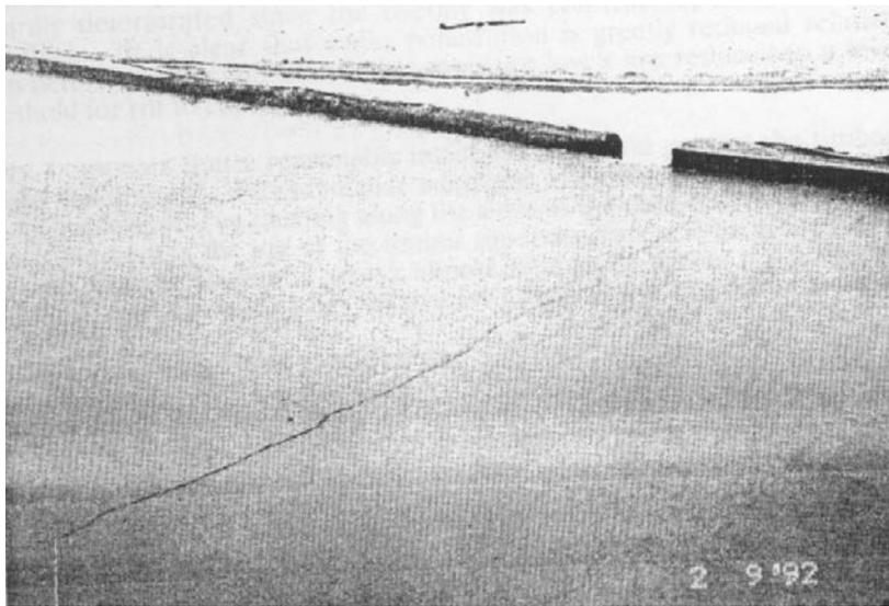
**Figure 6.3.3.3-1 Typical Transverse Cracking over Piers**
