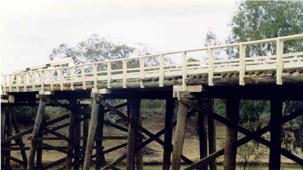
**Figure 6.2.1-1 Typical Round Timber Girder Bridge - Wakool River**
