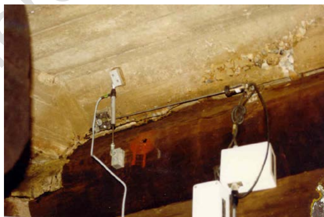
Figure 7.3.12-1 Instrumentation to Measure Slip and Separation
