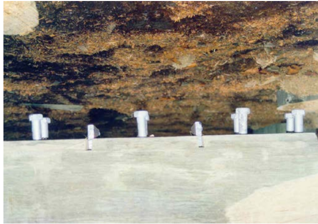
Figure 7. 2.4-2 Typical Shear Plates and Coach Screws
