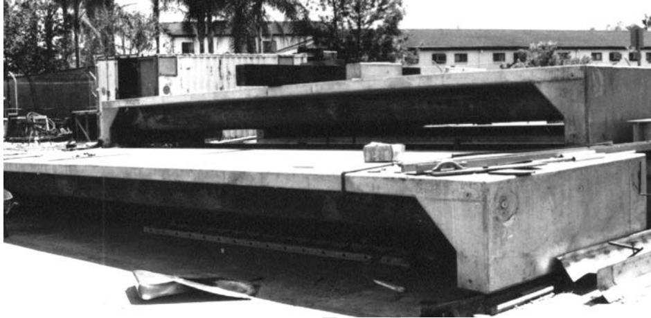
Figure 7.2-1 Deck Modules at RTA Fabrication Yard (Grafton)
