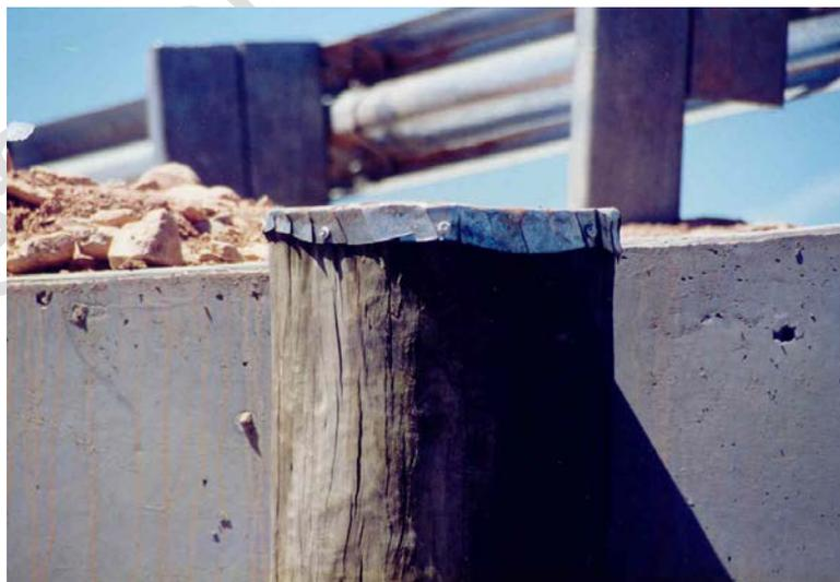
**Figure 8.3.2.2-2 Lignum Creek - End Capping of Timber Pile**
