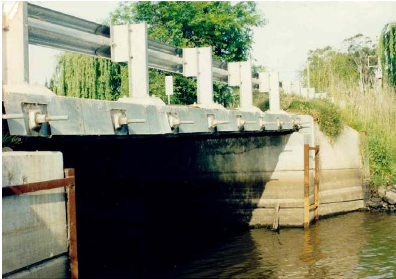
**Figure 8.3.2.2-3 Yarramundi Lagoon - Galvanised Edge Flashing**
