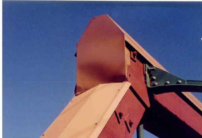
**Figure 8.3.2.2-1 Leycester Creek - Flashing over Truss Members**
