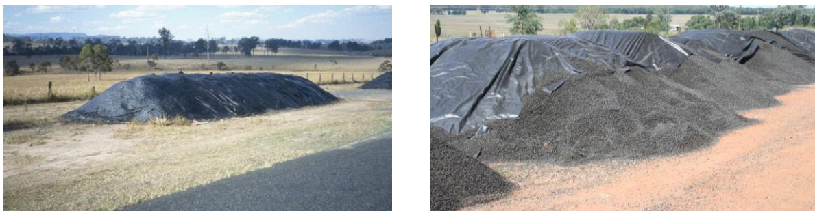
Figure NR107.2 – Covered Stockpiles
