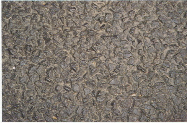
Matt seal (Note - polishing on tips of aggregate)
