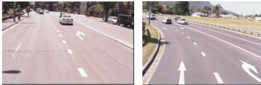
Figure 4.22: Continuity line at an edge of a portion of carriageway that is assigned to through traffic
