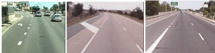
Figure 4.23: Continuity line intended to be crossed by traffic turning at an intersection, entering or exiting a motorway
