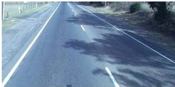
Figure 4.1: Dividing (separation) line on 2 lane road
