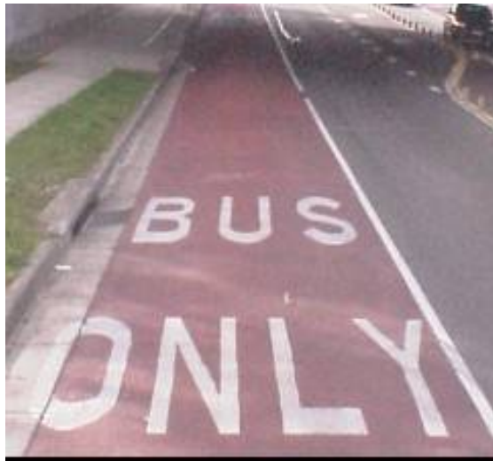
Figure 4.11: Bus Only Lane line (L6)
