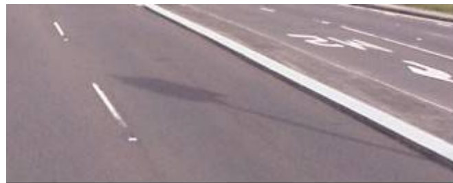
Figure 4.20: Edge line (E6) to mark incline surface of median
