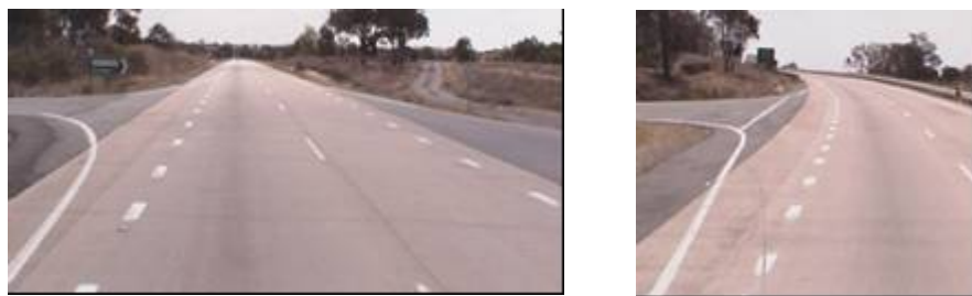
Figure 4.26: Continuity line to define the path of through traffic across an intersection
