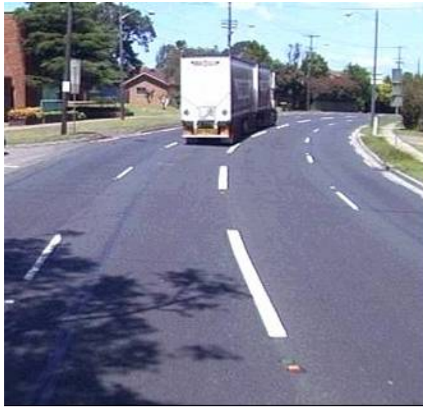
Figure 4.2: Dividing (separation) line on multi-lane road
