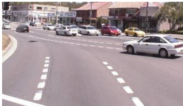
Figure 4.28: Turn Lines where there is more than one turning lane
