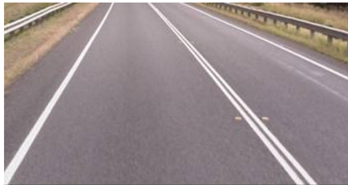
Figure 4.4: Dividing (barrier) line (two-way)
