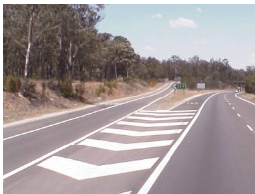
Figure 4.17: Edge Lines (E4) - Splayed approach
