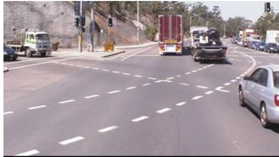
Figure 4.27: Turn Lines at a complex intersection
