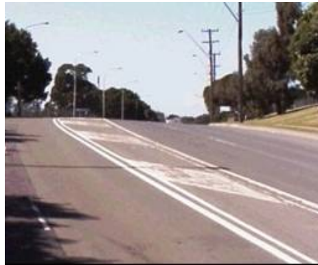
Figure 4.19: Double barrier lines to prohibit crossing
