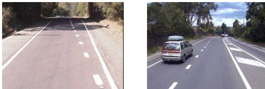
Figure 4.24: Continuity line intended to be crossed by traffic entering or leaving an auxiliary lane at start or finish
