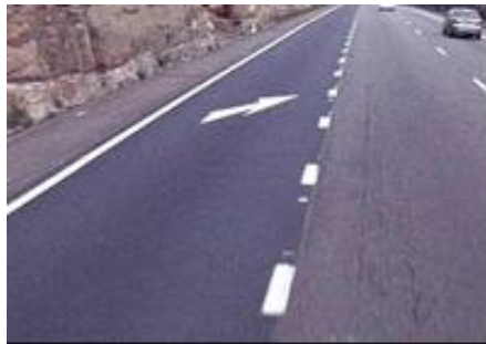
Figure 4.25: Continuity line where it is intended that the vehicle crossing should give way
