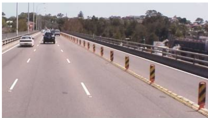
Figure 5.12: Enhanced lane separation devices (Collapsible delineator)
