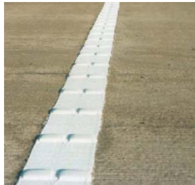
Figure 5.7: Raised ribs across profile linemarking
