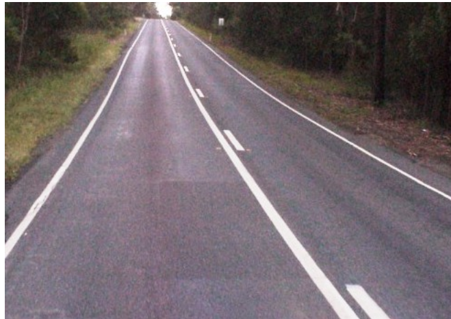
Figure 5.2: Enhanced dividing (barrier) line (BS1)
