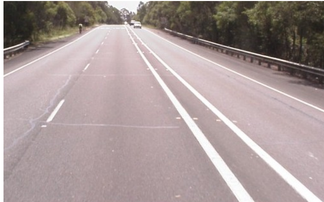
Figure 5.4: Enhanced dividing (barrier) line (BB2)
