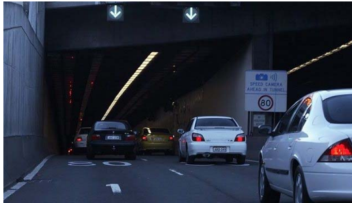
Figure 5.17: Application of Lane Usage Signs (LUS)
