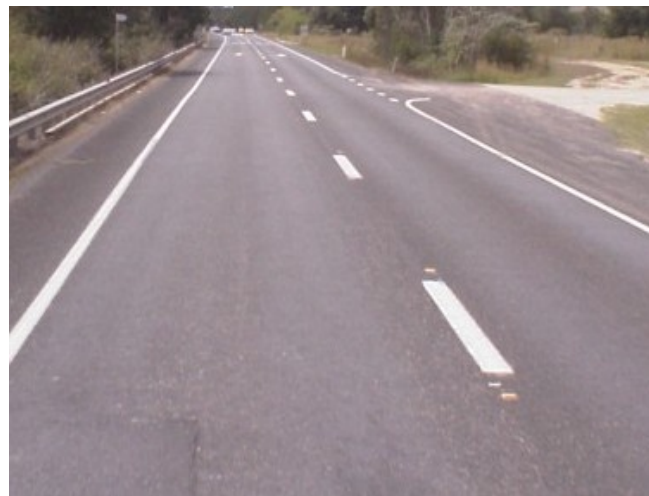
Figure 5.1: Enhanced dividing (separation) line (S3)
