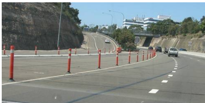
Figure 5.13: Enhanced lane separation devices (Flexible bollards)
