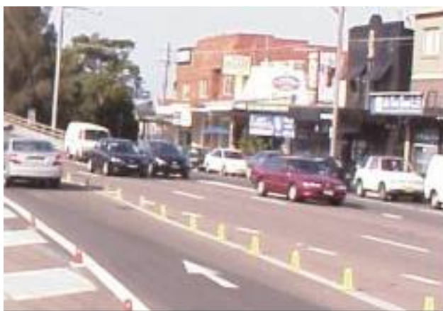
Figure 5.11: Enhanced lane separation devices (Pavement flaps)
