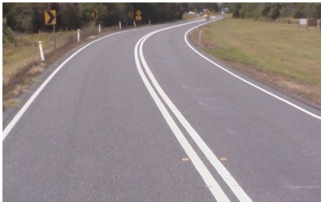
Figure 5.3: Enhanced dividing (barrier) line (BB1)
