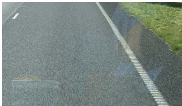
Figure 5.9: Type B Profile linemarking
