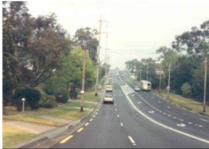
Figure 2.6: Short range delineation - pavement markings and raised pavement markers
