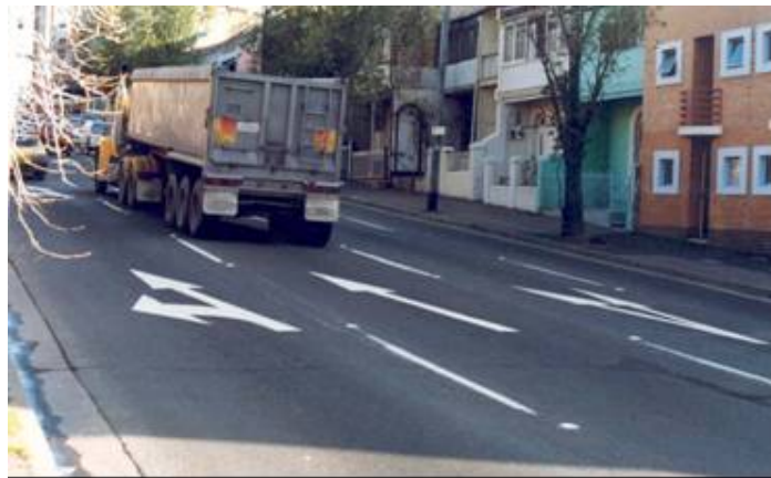
Figure 2.1: Delineation function - position and movement of traffic
