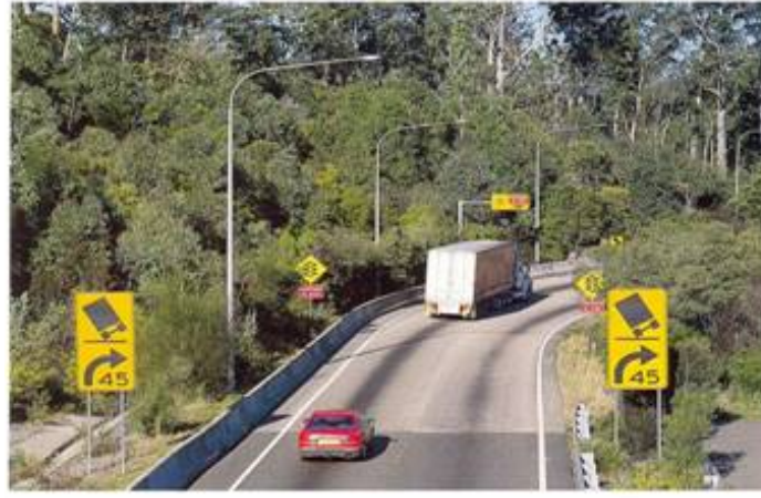
Figure 2.5: Delineation function - Identifying potentially hazardous situations
