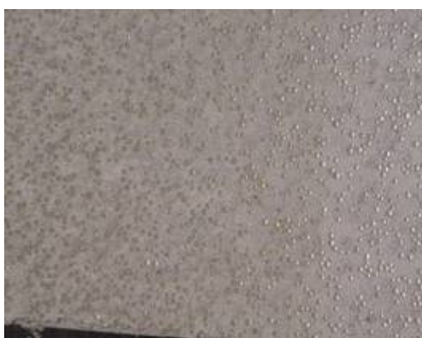
Figure 2.9: Glass beads embedded in pavement marking material
