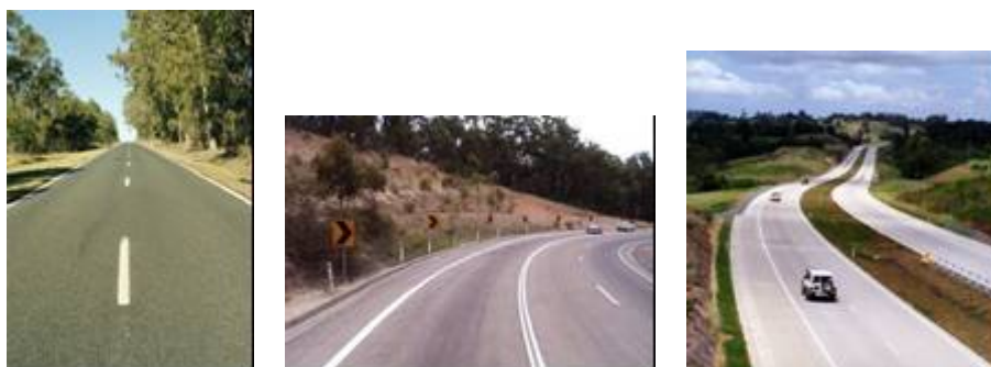
Figure 2.11: Road geometry and types of pavement surface affect selection of delineation devices
