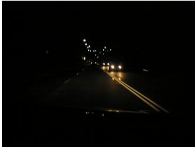
Figure 3.3: Limitations of pavement marking - wet roads
