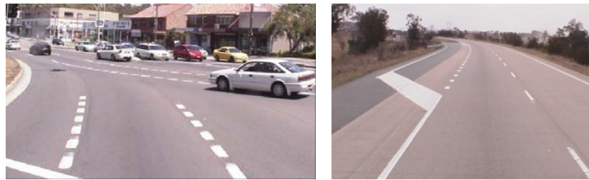
Figure 3.1: Pavement Markings providing positive guidance
