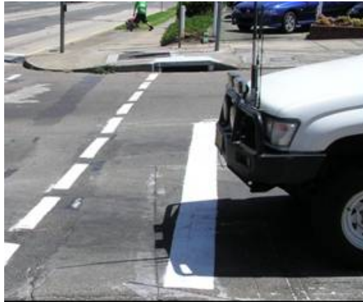
Figure 6.1: Stop line at signals
