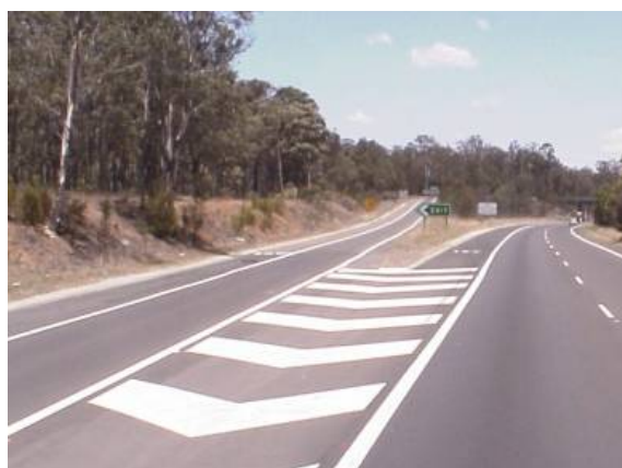
Figure 8.1: Splayed approach with chevron markings
