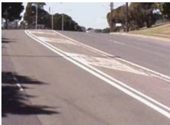
Figure 8.7: Example of painted median where driving on or crossing is prohibited
