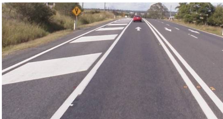
Figure 8.4: Example of diagonal marking on shoulders
