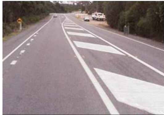
Figure 8.2: Painted Median with diagonal markings
