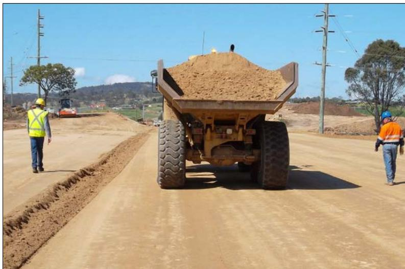
**Figure 14: Proof rolling being carried out using a fully laden gravel truck**
