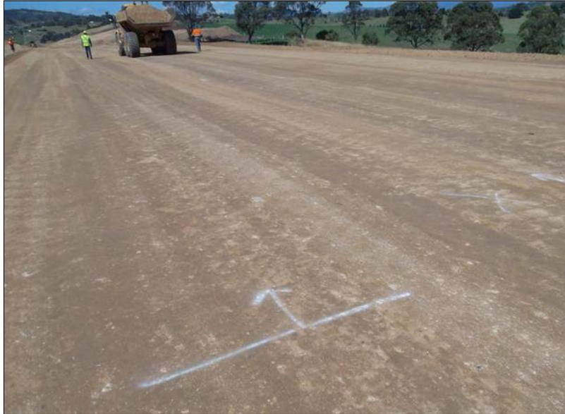
**Figure 15: Areas marked for rehabilitation after failing proof rolling**
