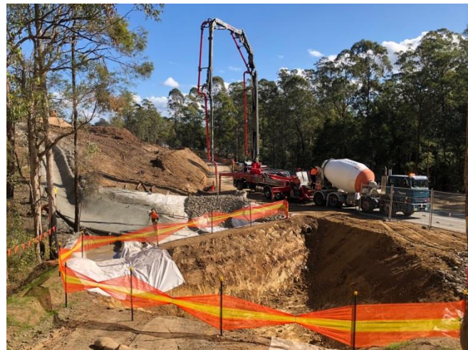
Above: Placing concrete to line a new catch drain
