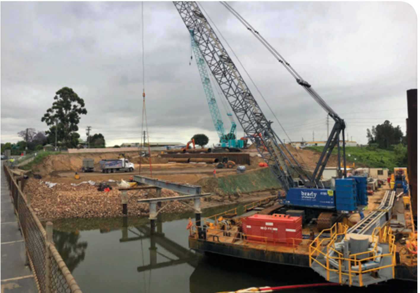
Work on the northern side of the river and the barge
