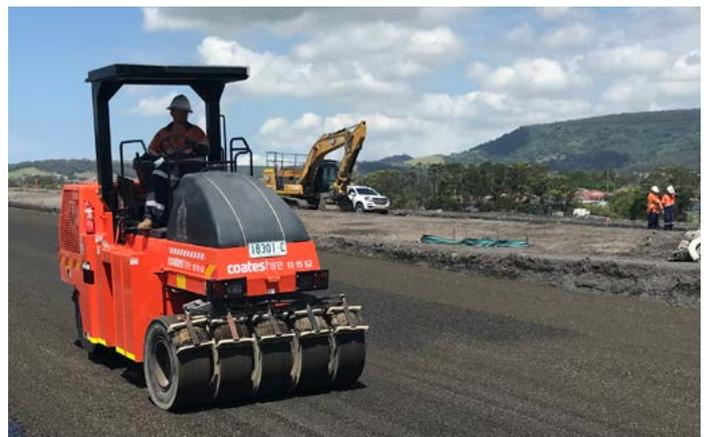
Pavement base layer being placed on the new motorway north of Tongarra Road
