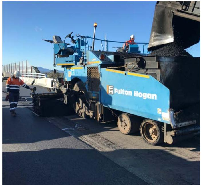
Recycled crushed glass being used in asphalt at Croome Road
