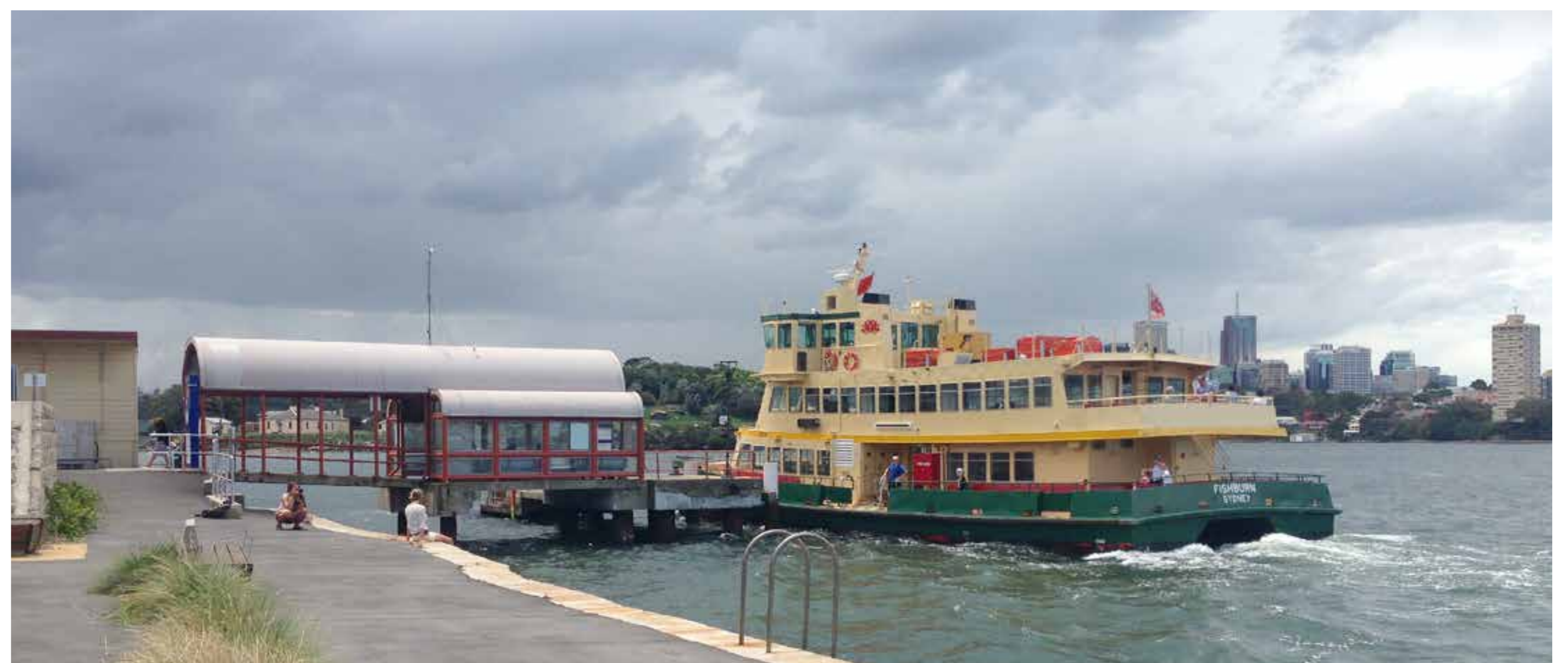
Existing Balmain East Wharf viewed from the land.
