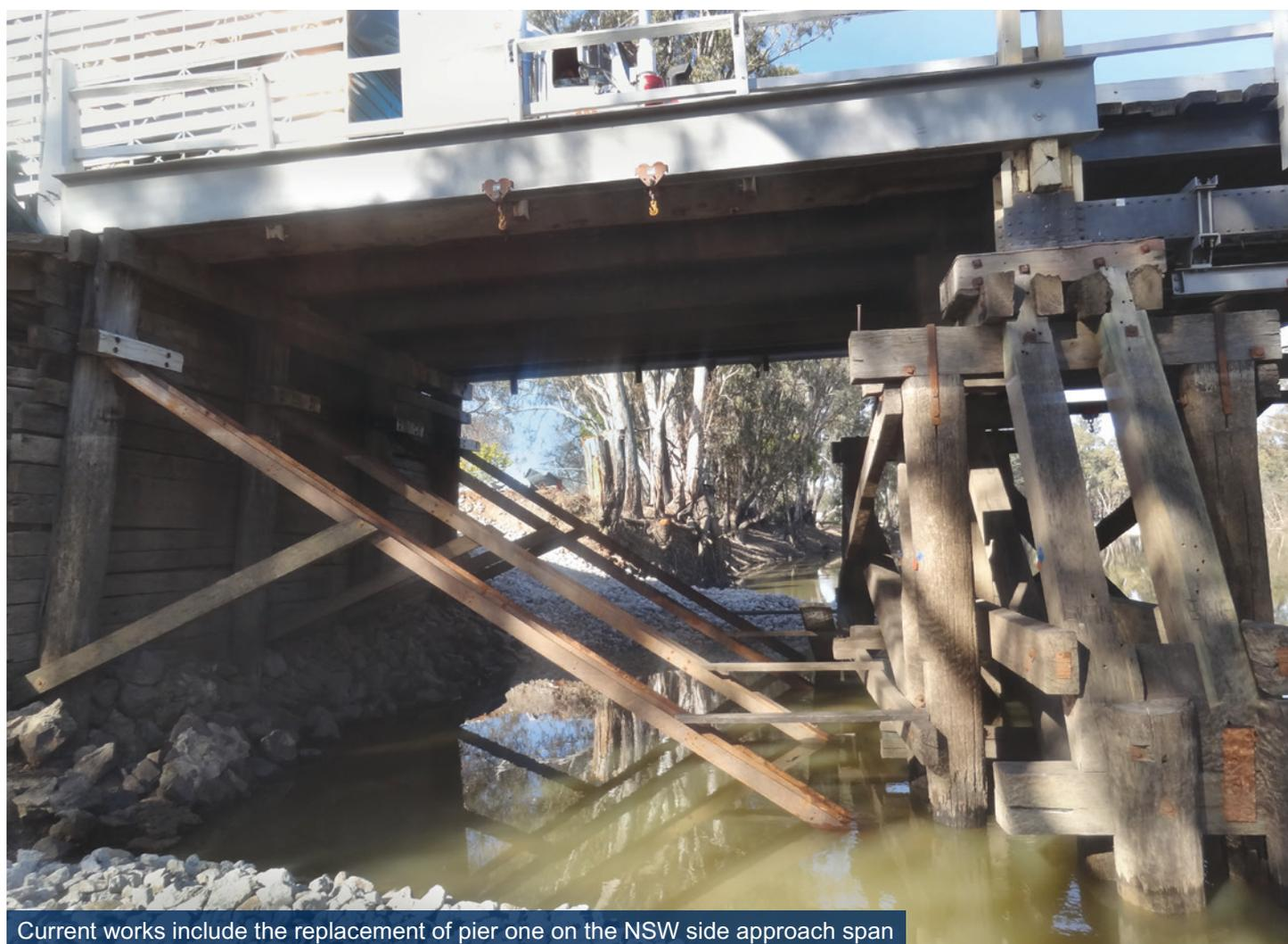
Current works include the replacement of pier one on the NSW side approach span
