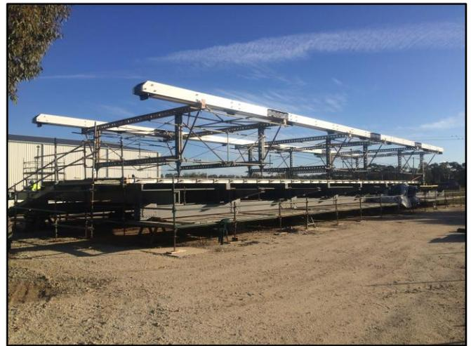
Truss span two being assembled in the Koondrook site compound.
