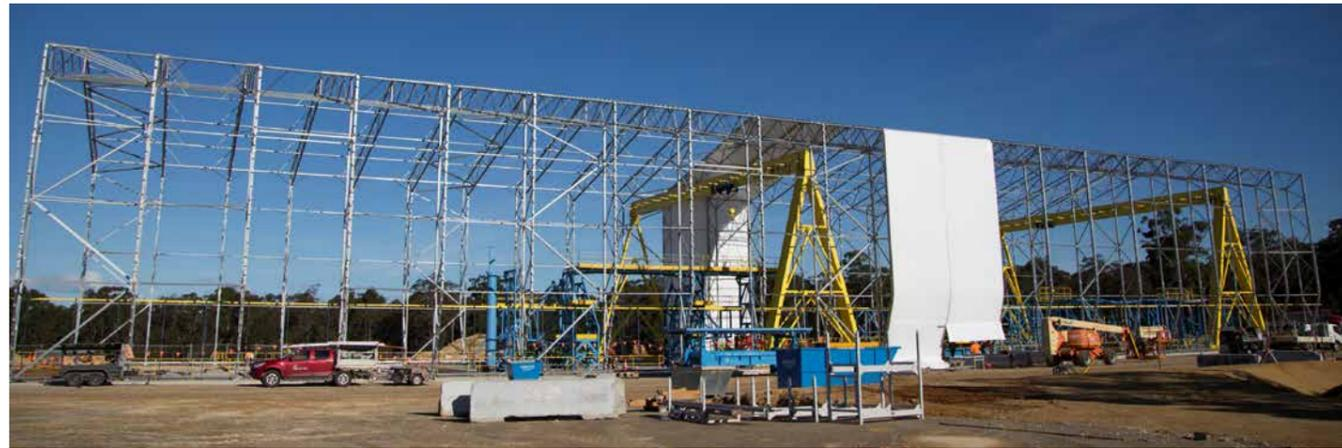
Special polyethylene high tensile sheets are being pulled over the roof of the pre-cast production shed in readiness for segment production in July.
