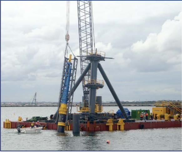
A typical barge and crane set up for piling work
