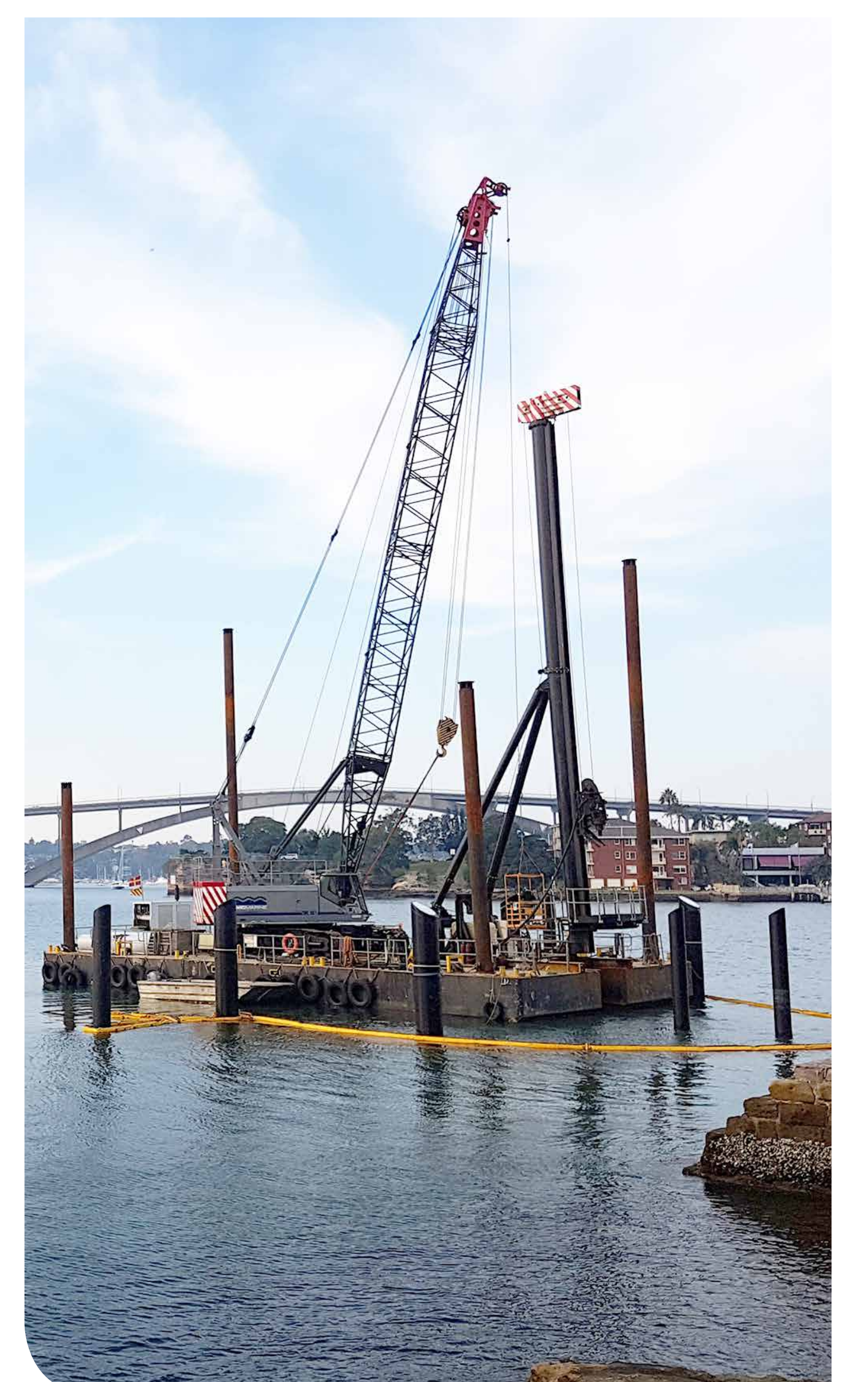
Barge-mounted crane at Chiswick
