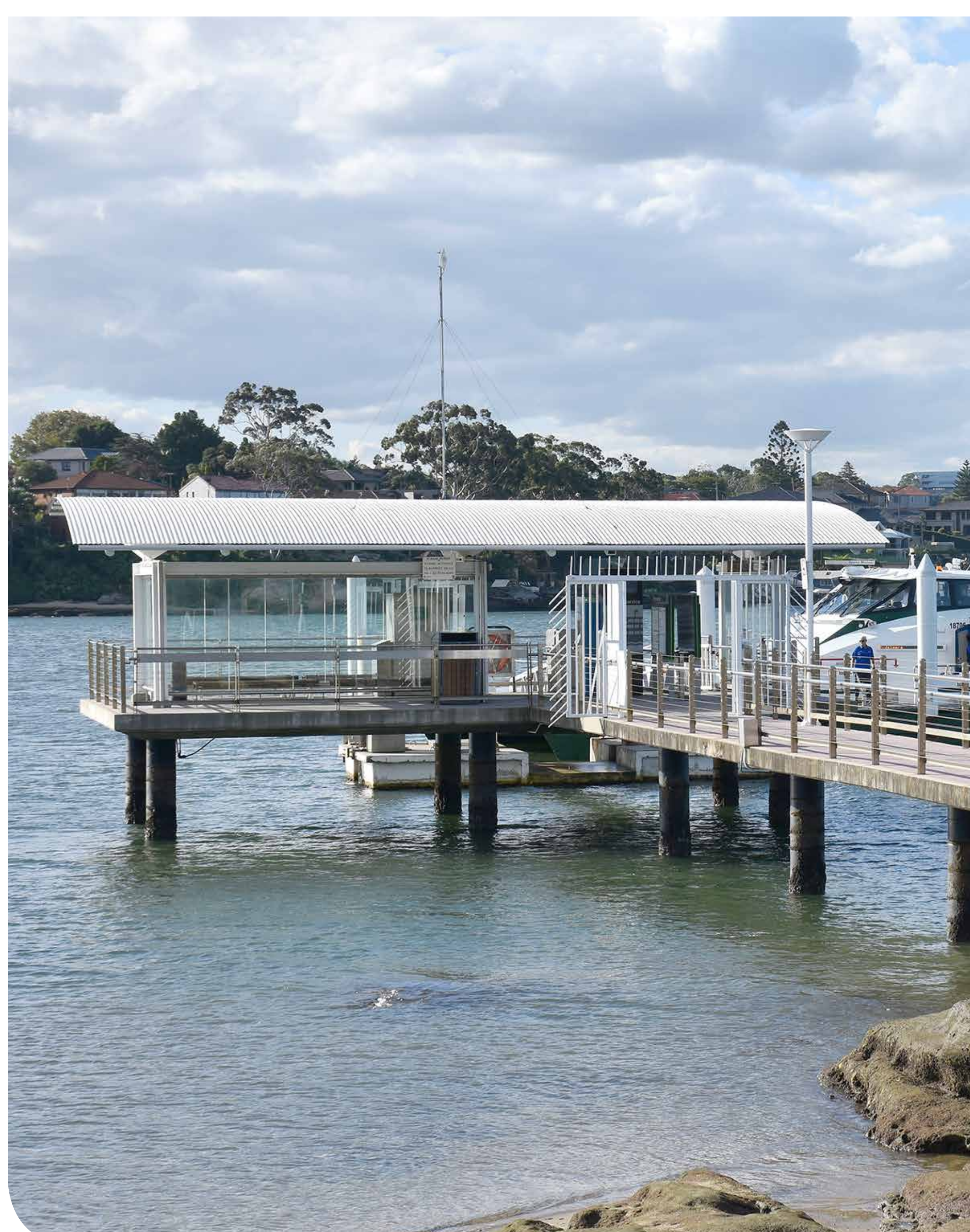
The existing wharf
