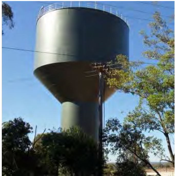
Figure 5-2 New Sydney Water tower at Zouch Rd
