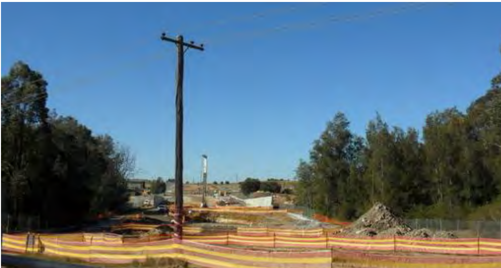
Figure 5-1 Glenfield to Leppington Rail Line under construction
