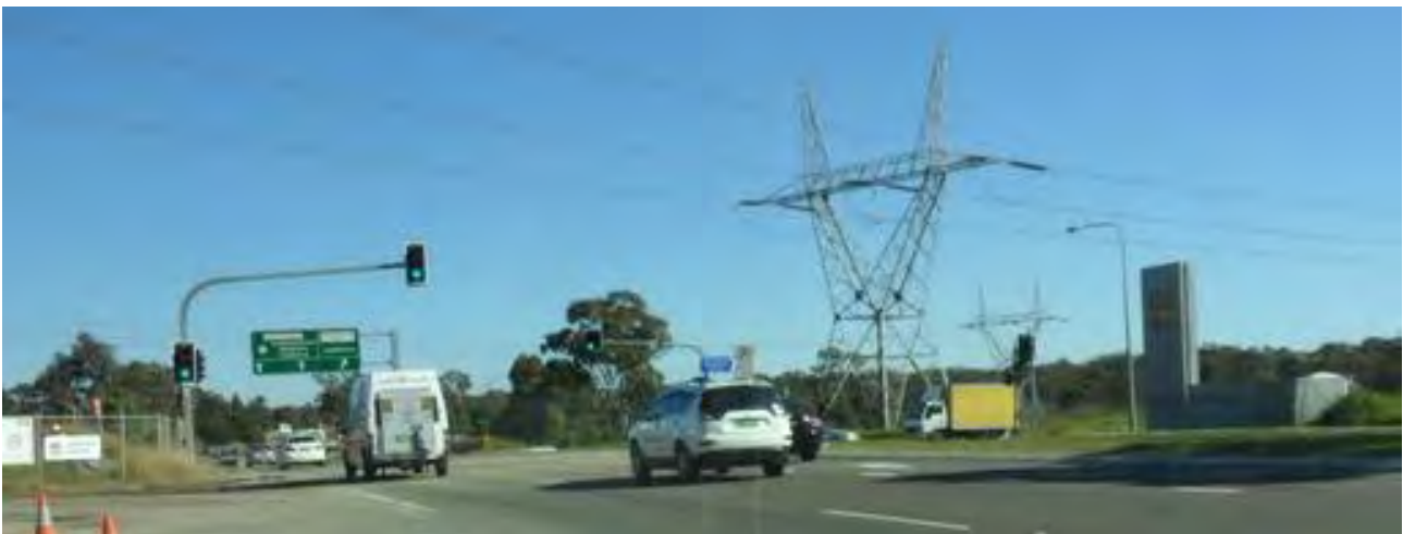
Figure 5-4 TransGrid transmission towers at Beech Rd
