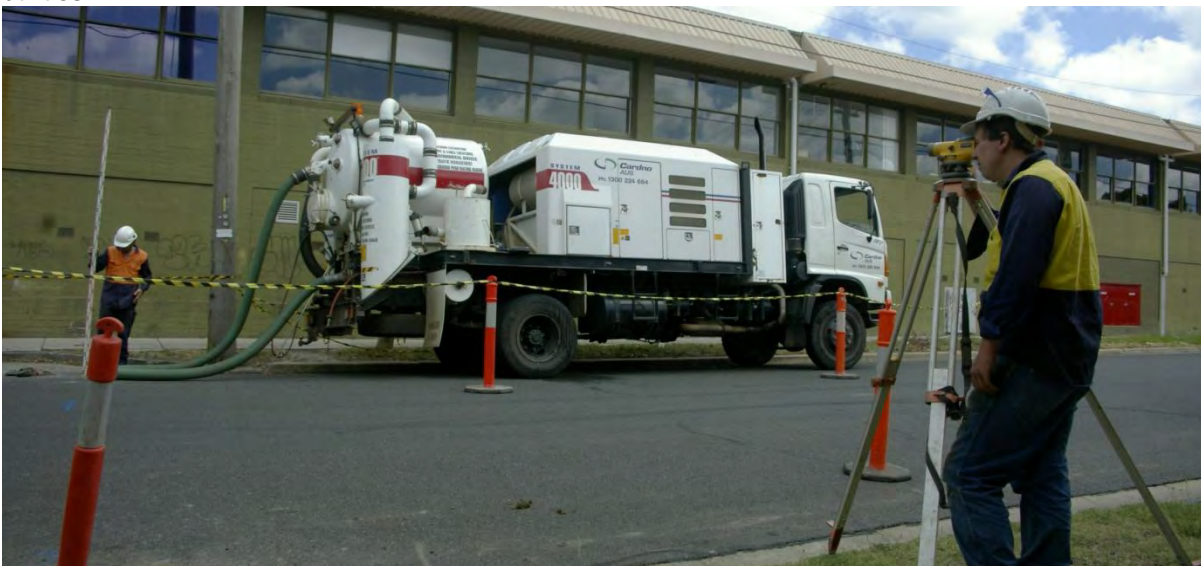
Figure 7-2 Vacuum truck potholing to physically locate service
