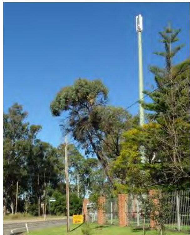
Figure 5-3 Vodafone base station at Zouch Rd
