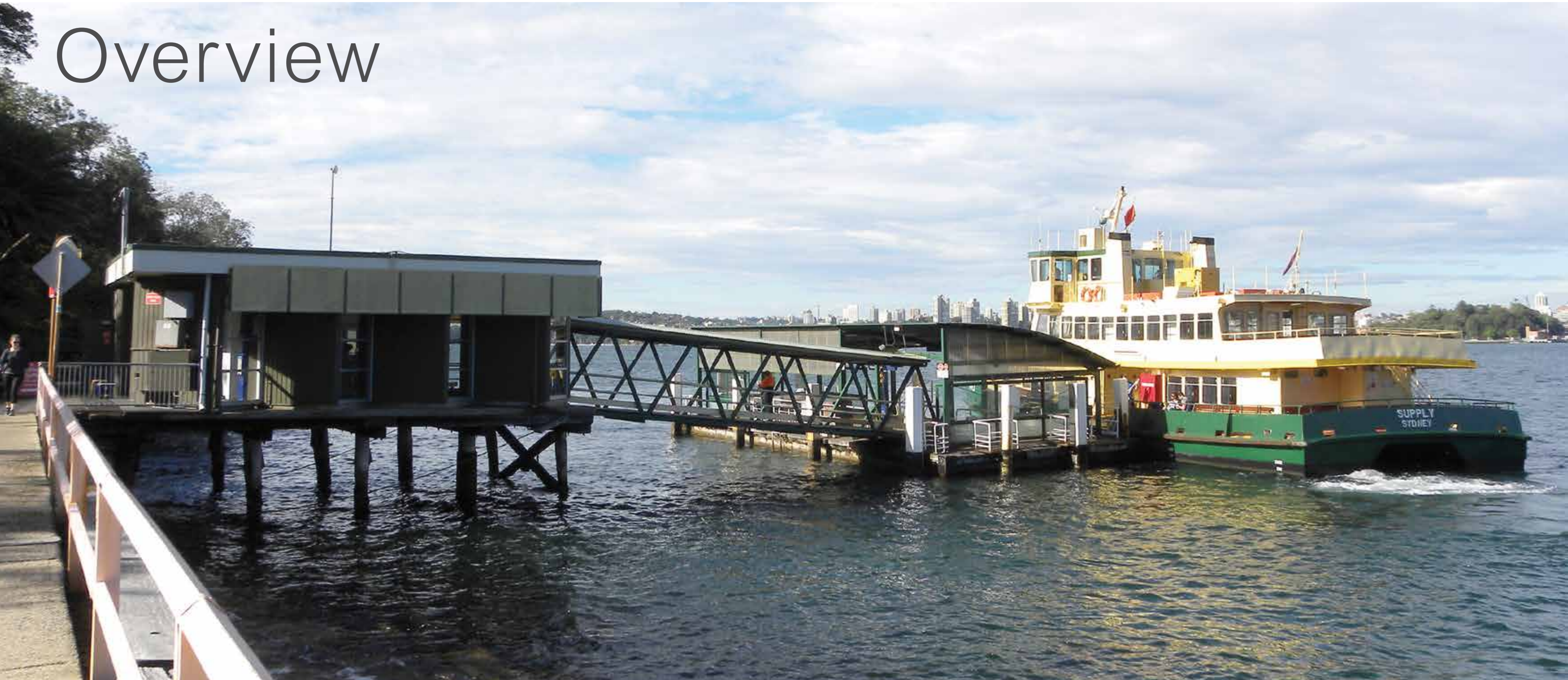
Existing Cremorne Point Wharf.
