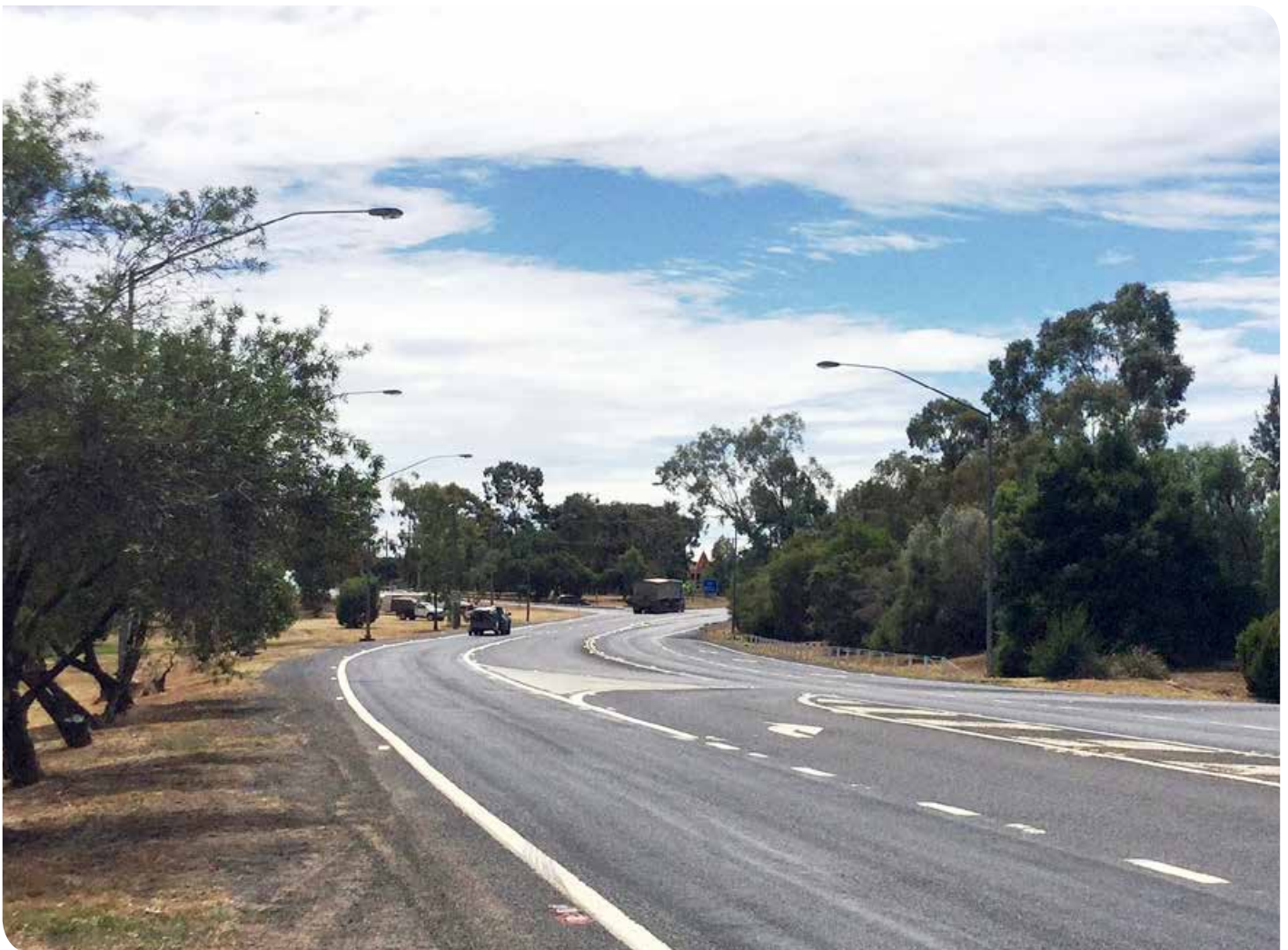
View looking towards the Minore Road and Newell Highway intersection
