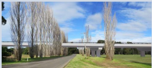
Berry Bridge will consist of 228 beams (girders), each weighing up to 50 tonnes and 33 metres in length.
