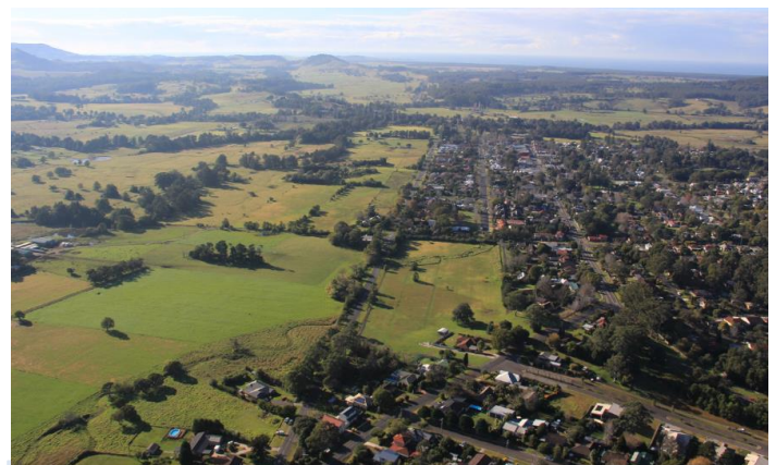
Major construction has started on the Foxground and Berry bypass with work to be completed in mid 2018, weather permitting.
