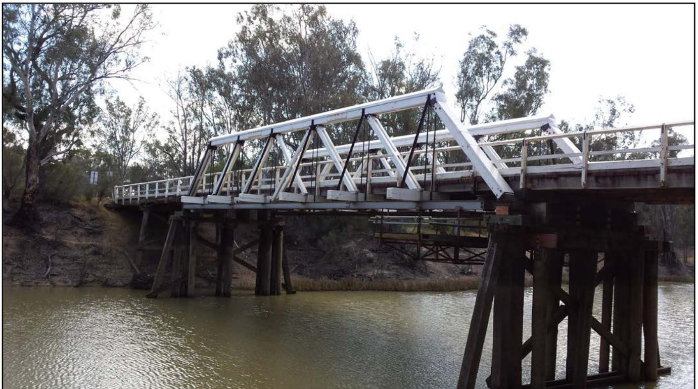
**Gee Gee Bridge was built in 1929 and is a Dare type timber truss bridge.**
