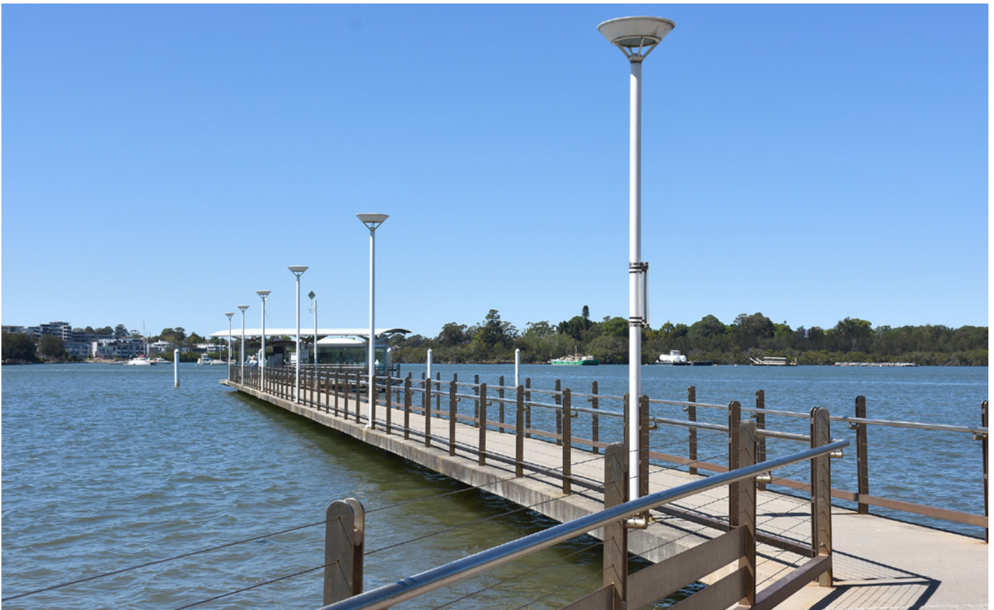
The existing Kissing Point Wharf viewed from land
