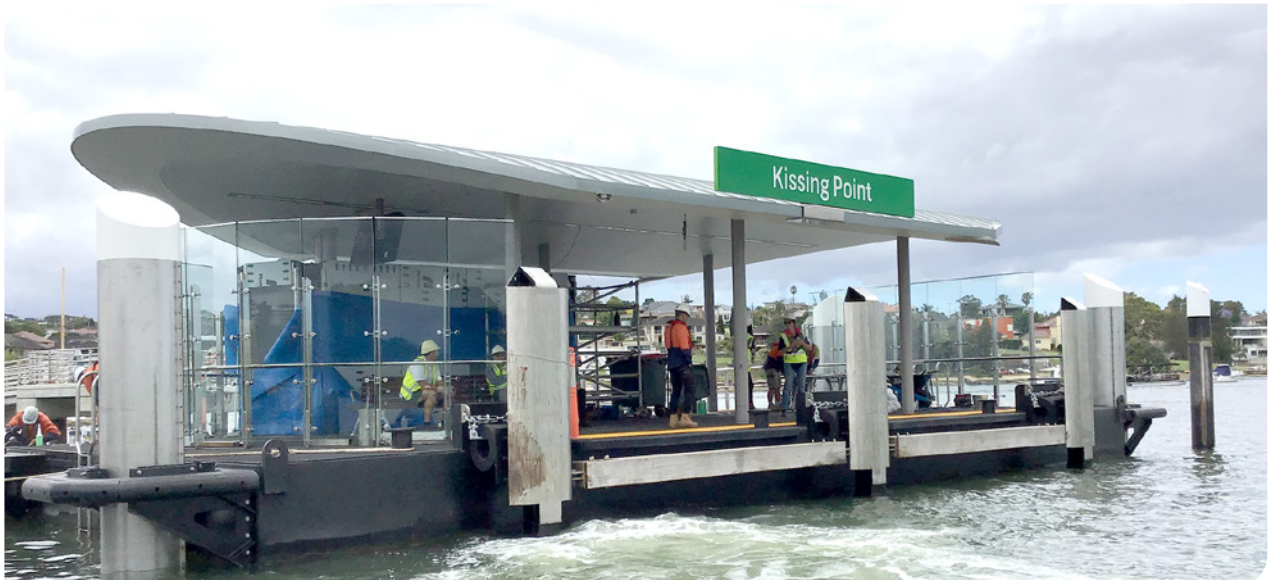
Kissing Point Wharf construction nearing completion
