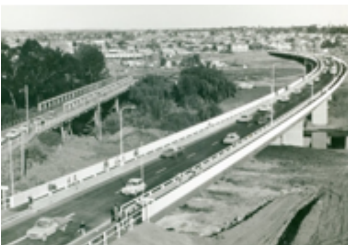
The bridge in 1969
