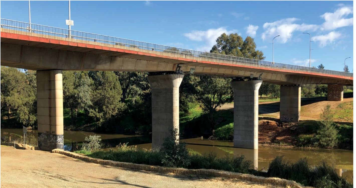
Two new strengthening piers on the LH Ford Bridge, Dubbo
