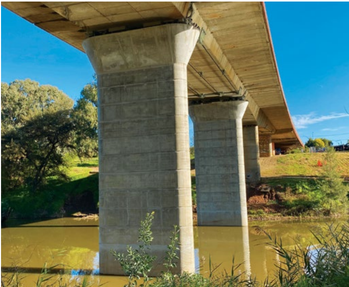
Work completed under the bridge
