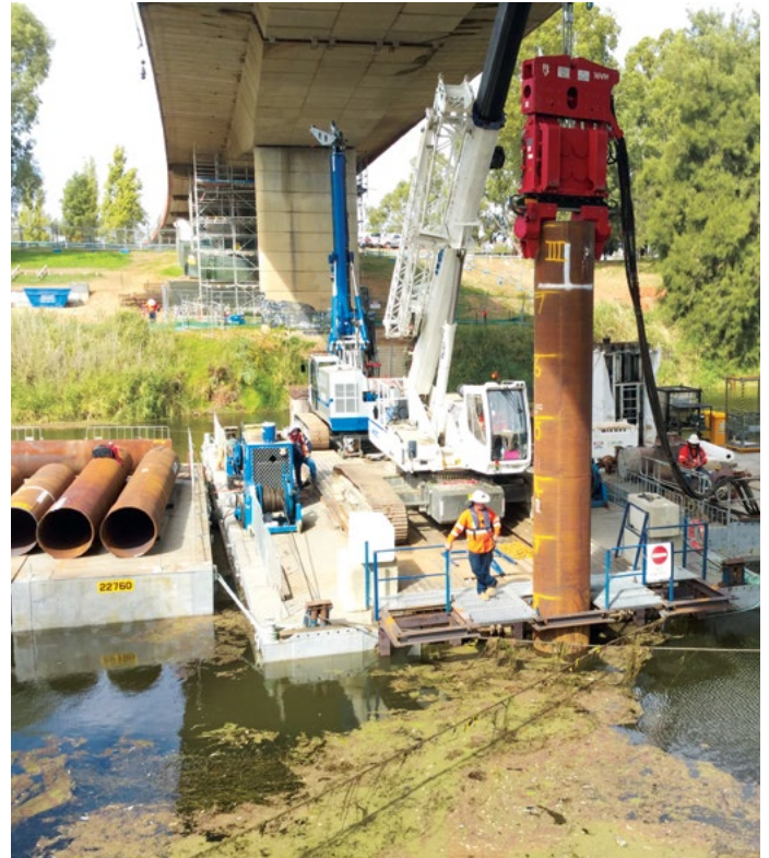
Driving in casings for the piles, part of pier construction
