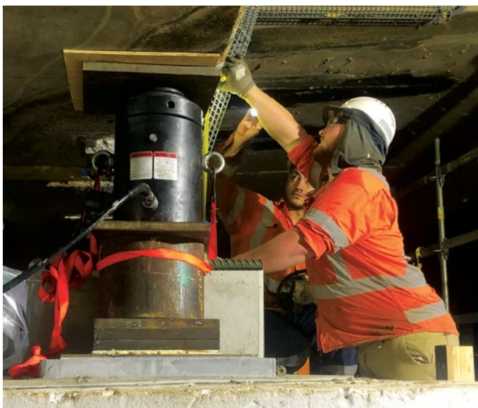
Connecting the new piers to the bridge
