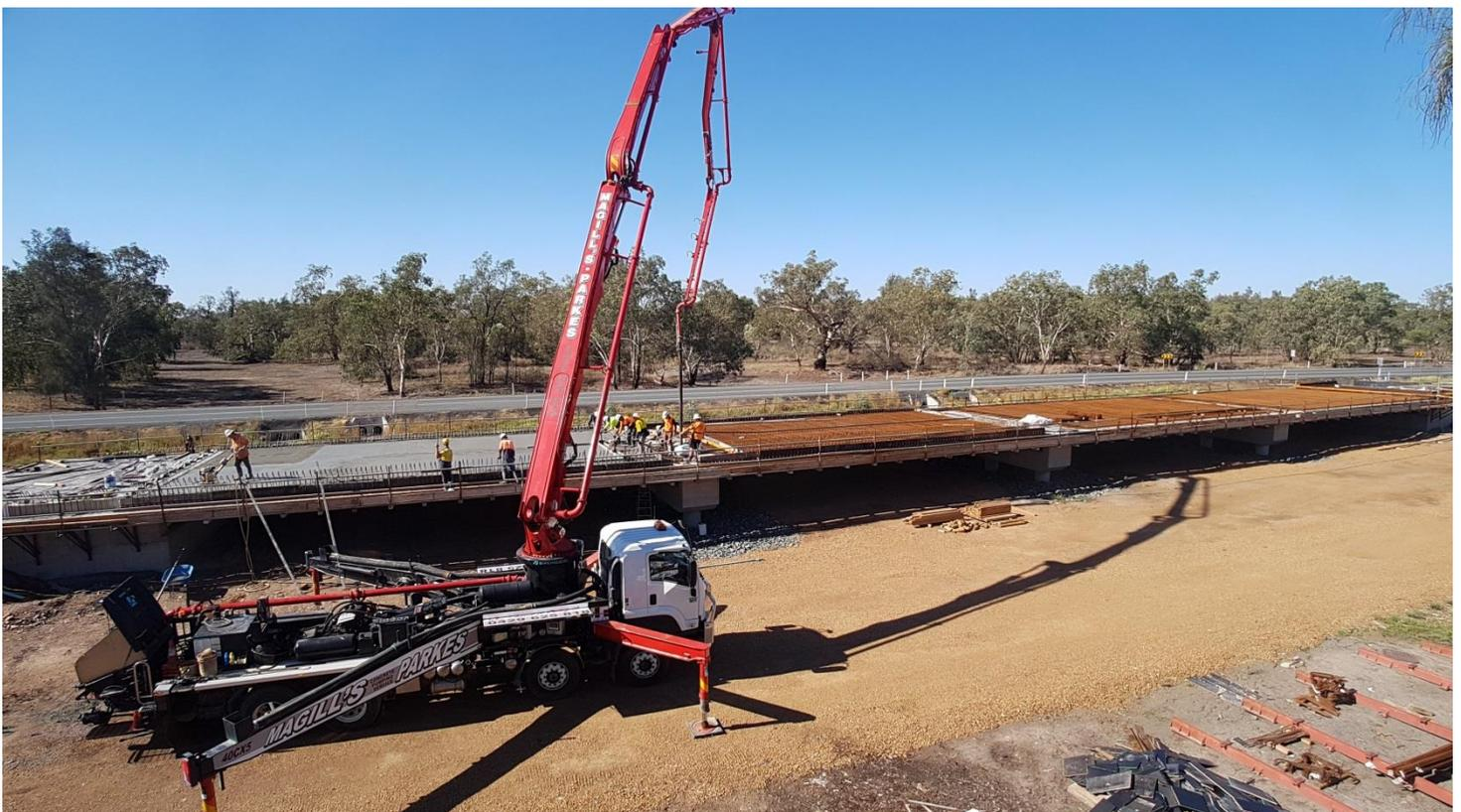
Concrete being poured to form the Lignum Creek Bridge deck
