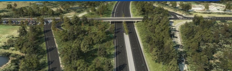
Artist impression of Warnervale Interchange, now completed as part of the M1 Upgrade between Tuggerah and Doyalson
