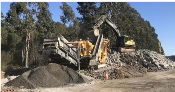
Concrete crushing in progress
