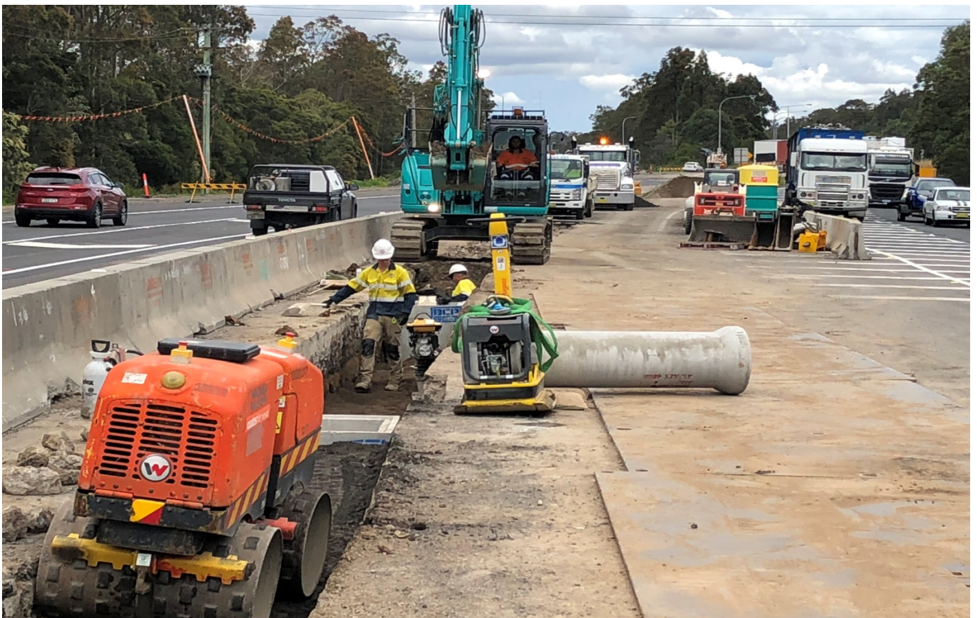
Digging pits and laying stormwater pipes
