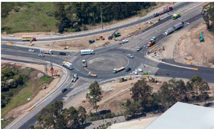
October 2018: M1 Upgrade at Weakleys Drive and John Renshaw Drive intersection
