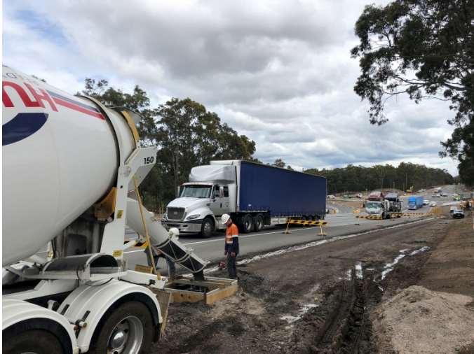
Pouring concrete footings for street light poles
