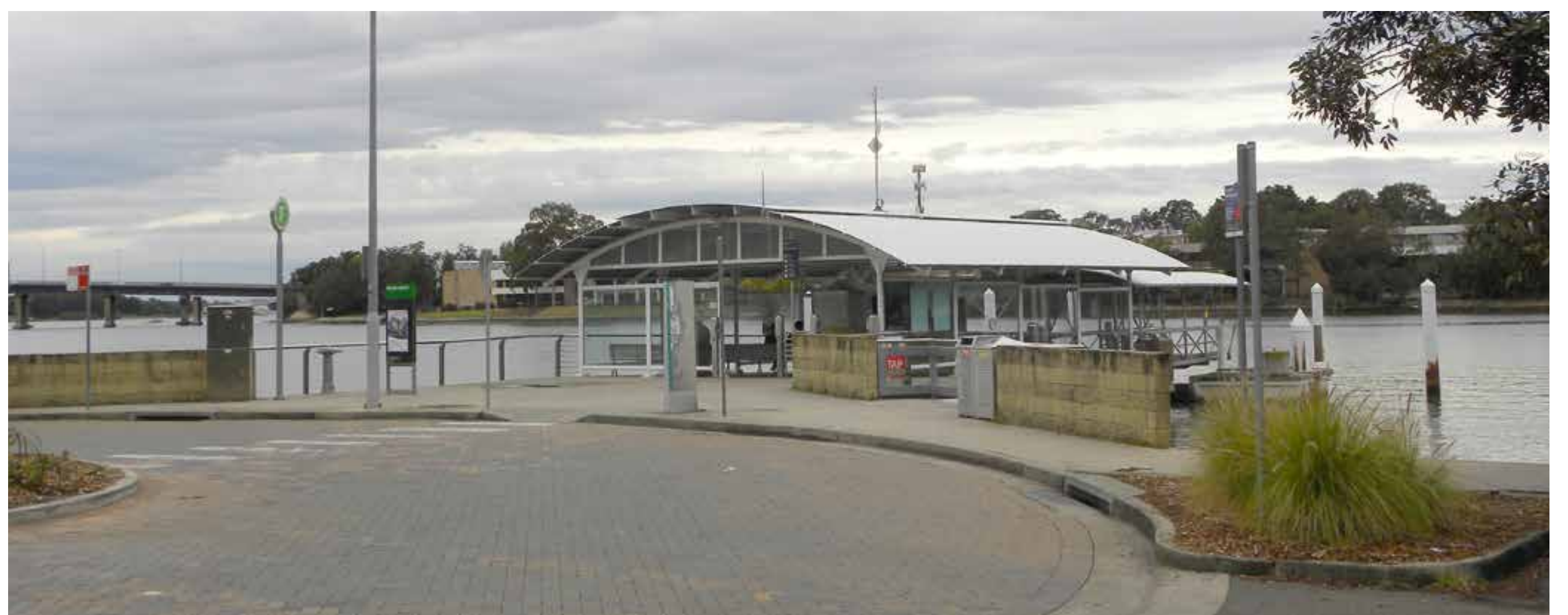
The existing Meadowbank Wharf and interchange
