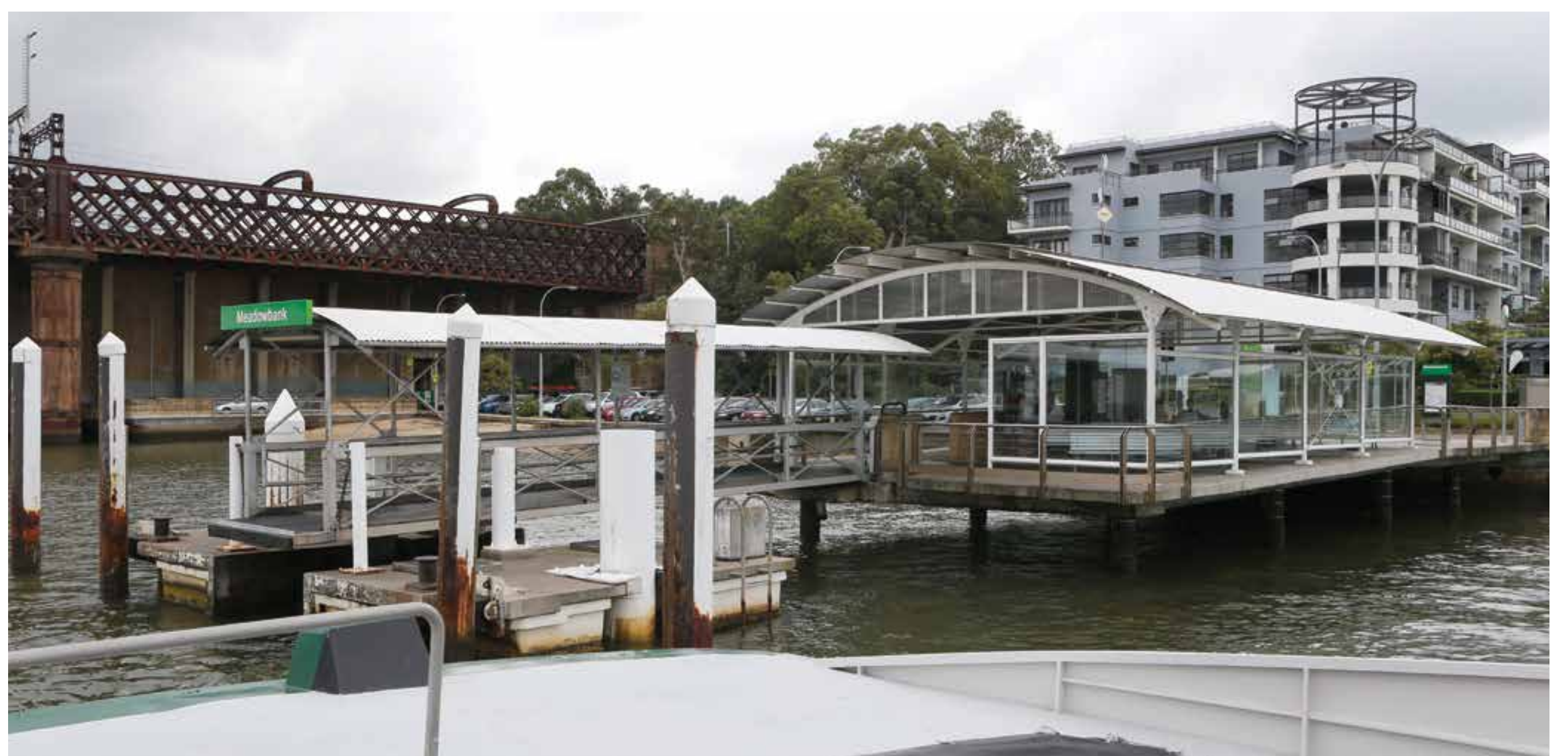
The existing Meadowbank Wharf viewed from the water
