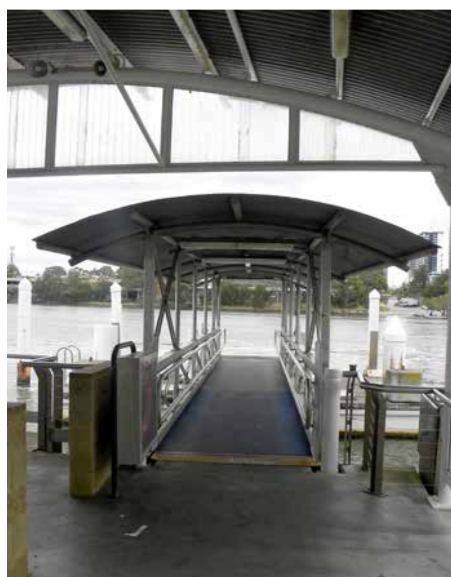
The existing Meadowbank Wharf and interchange
