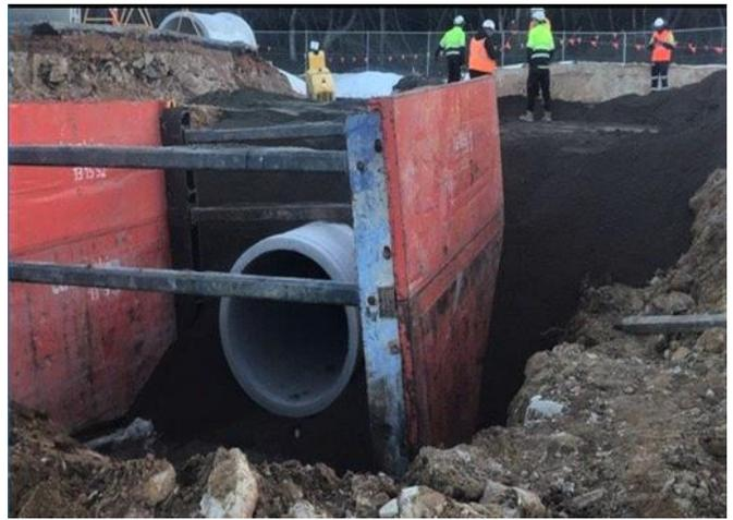
One of the major deep stormwater drainage crossings installed during the 56 hour road closure – 1650mm pipe
