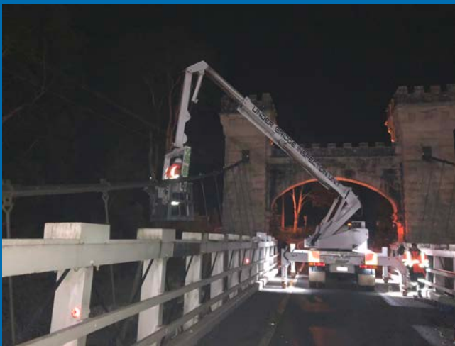
Repair work on Hampden Bridge during bridge closure, May 2018
