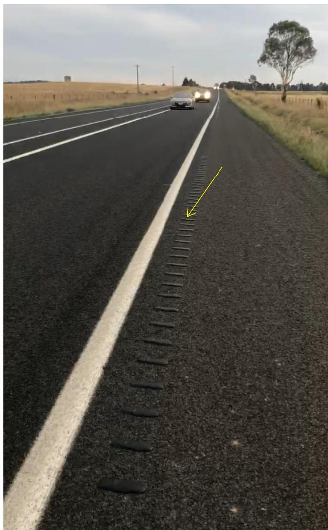
*Audio tactile line marking applied at 200mm offset from edge lines and wide centreline*
