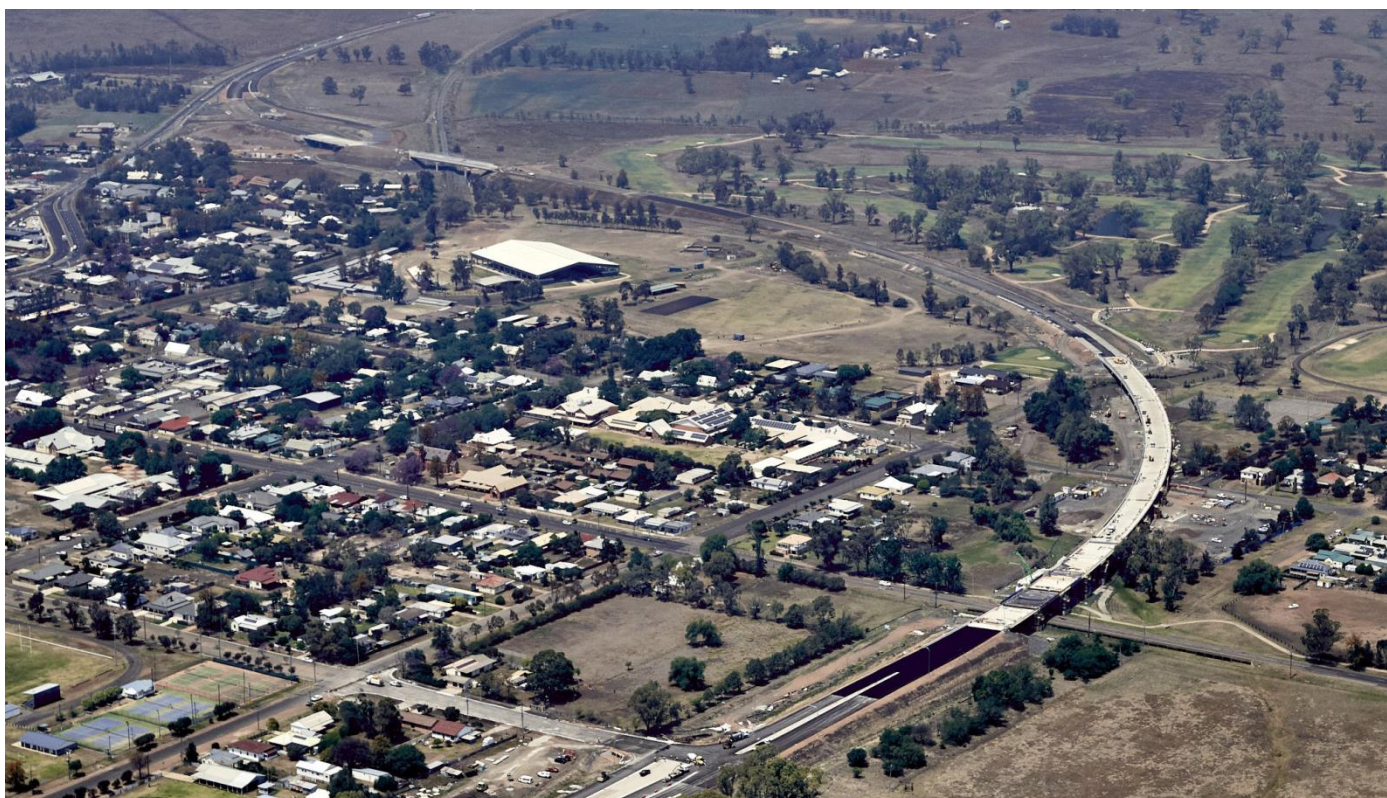
Aerial view looking south in late October showing the completed concrete deck of the bridge over Parsons Gully
