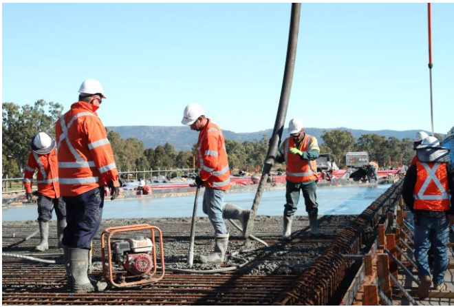
Workers placing concrete on the rail bridge deck
