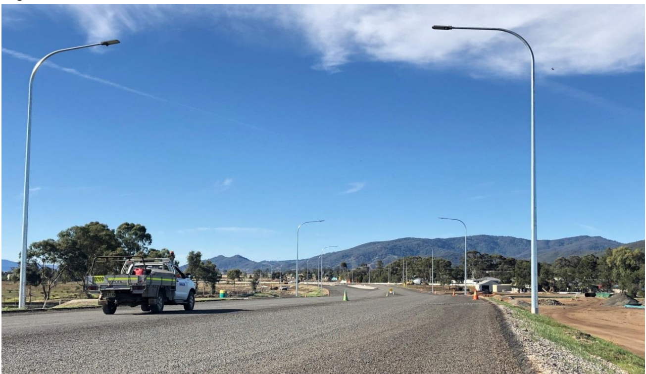
Street lights at the northern bypass intersection. We use energy-saving and efficient LED lights, which will focus light onto the bypass
