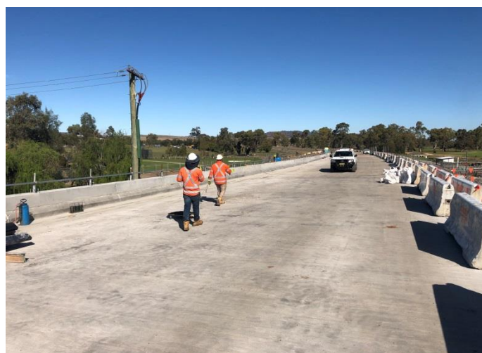
Concrete deck at southern end of the bridge over Parsons Gully
