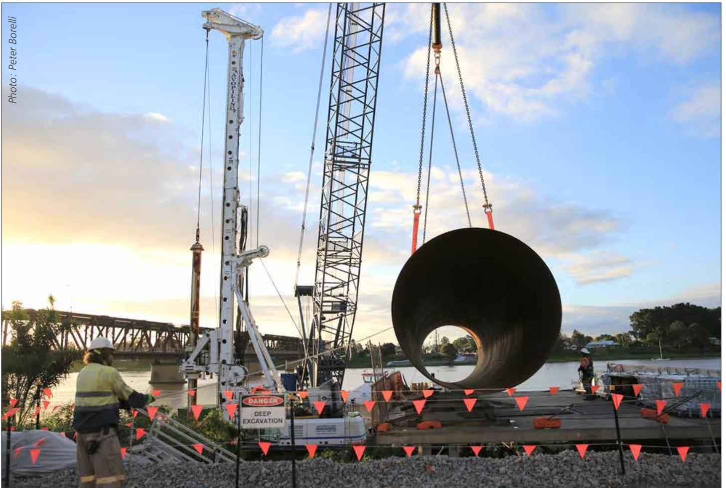
A steel casing for a marine pile being lifted by the crane on the southern embankment
