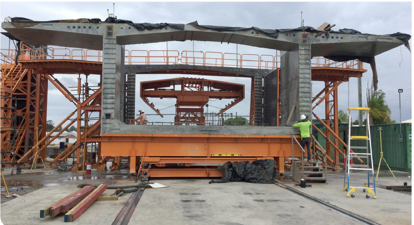
First concrete bridge segment poured at the pre-cast facility in January
