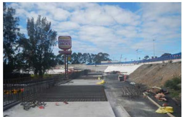
Construction of retaining wall behind Hungry Jacks
