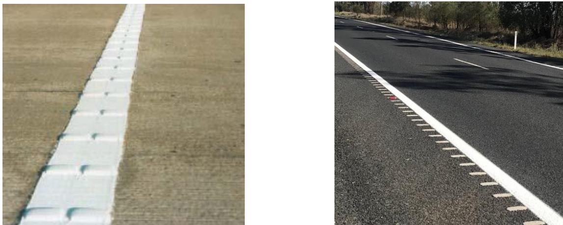
Figure 2 – Examples of ATLM installation.
