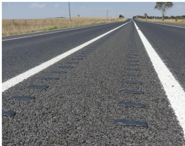
Figure 7 – Example of black ATLM rib placement for wide centreline treatments
