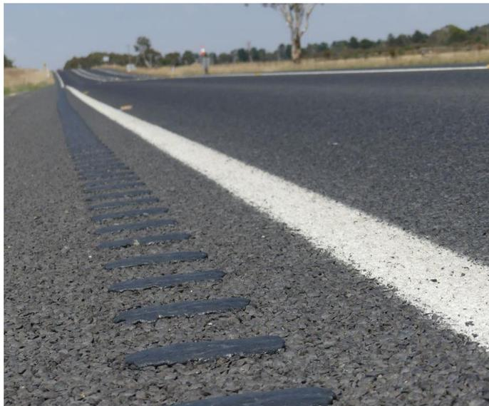
Figure 4 Example of installed black ATLM raised ribs on edge lines on rural high speed roads
