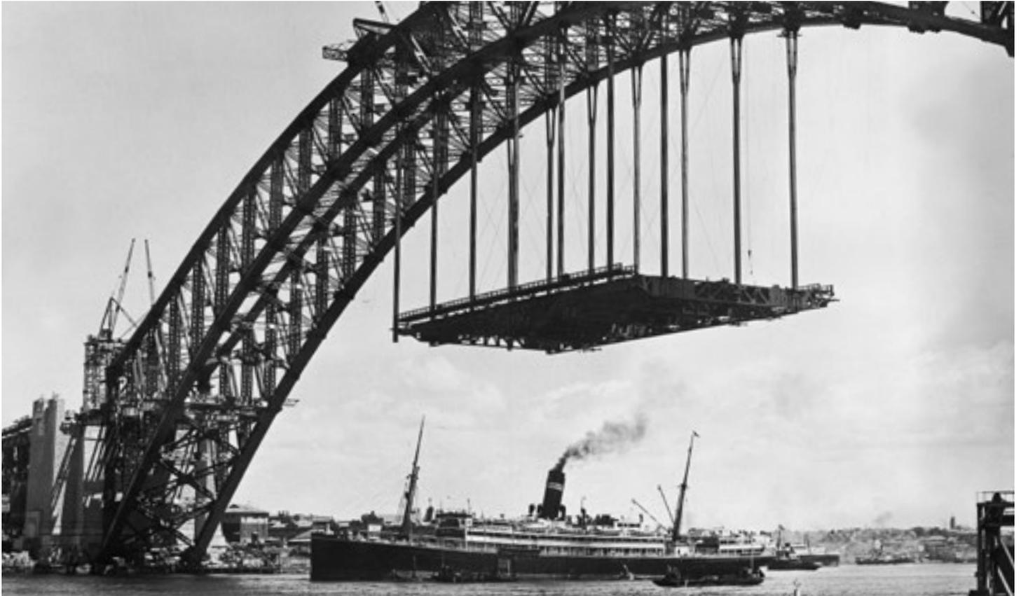
Decking suspended from the completed arch while a steamship passes underneath.
