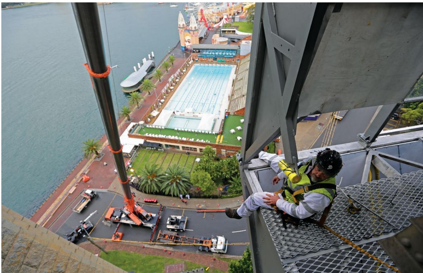
Workers installing the containment structure for the repainting program
